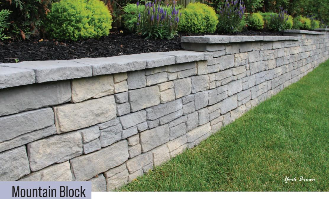
Mountain Block's single-sided face provides a unique stone texture with its 4" x 12" wall face. Solid block makes this system structurally sound for walls with a maximum height of 36". Its organic design stylishly connects your home to its natural surroundings. Nicolock's Rockface Multi-Cap can be used to add the finishing touch to a great outdoor setting.
